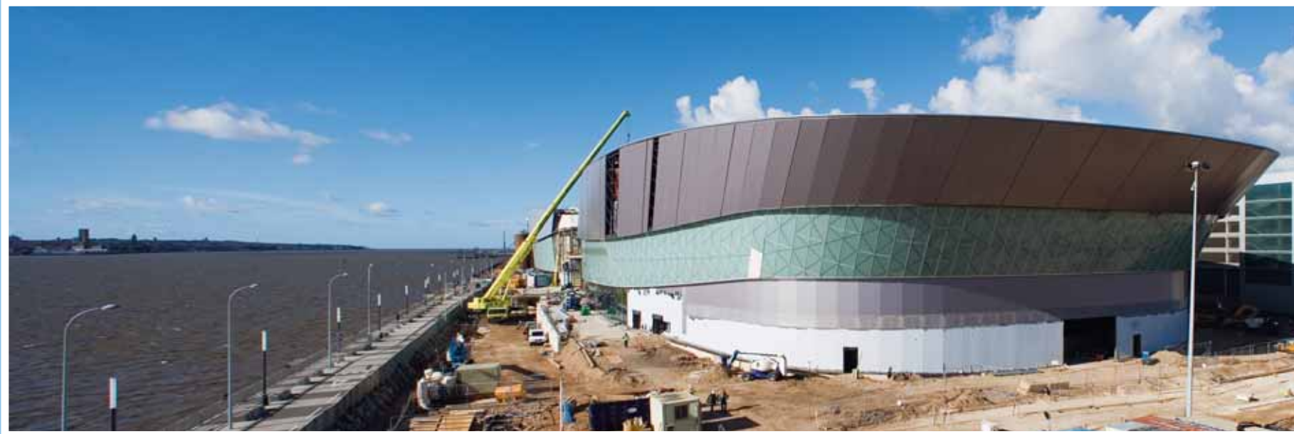
Construction of Arena and Convention Centre Liverpool, 2007
