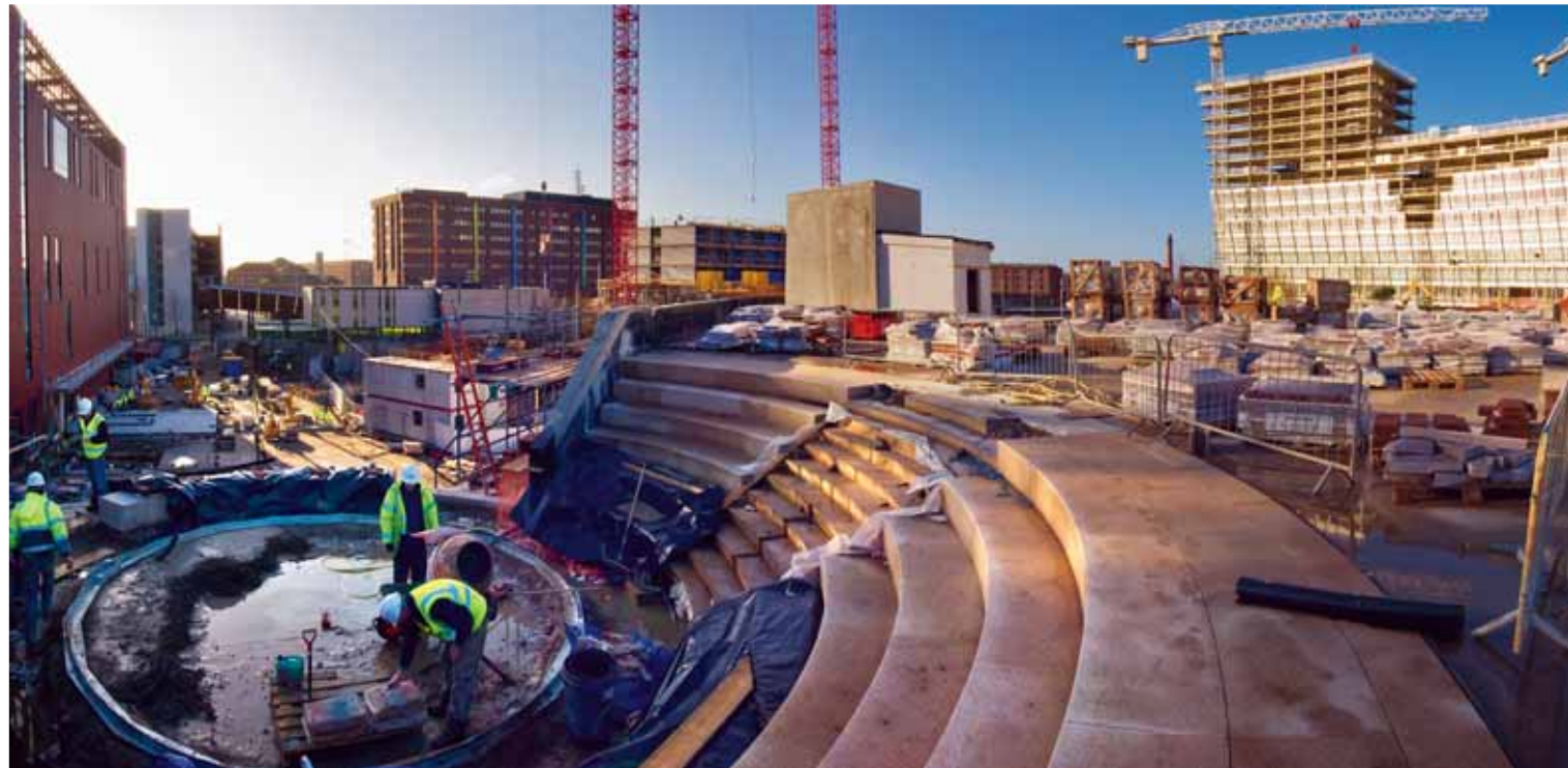
Construction work at Liverpool One, 2007
