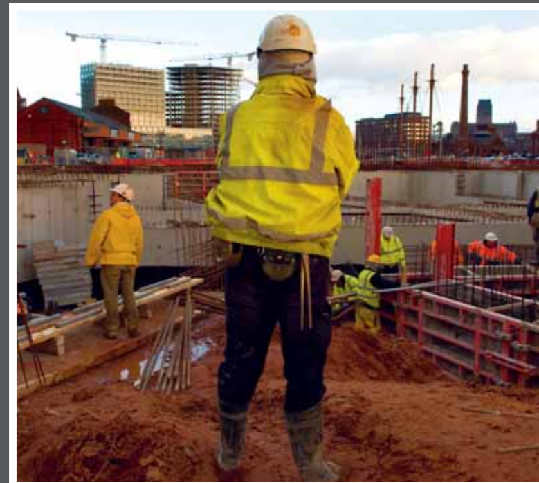
Construction of the Museum of Liverpool
