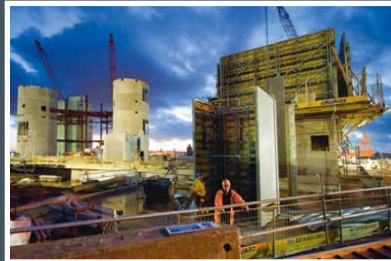
Construction of the Museum of Liverpool, 2007
