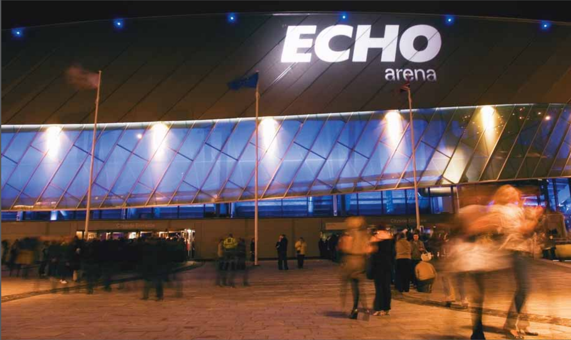
Liverpool Echo Arena at Kings Waterfront, 2008
