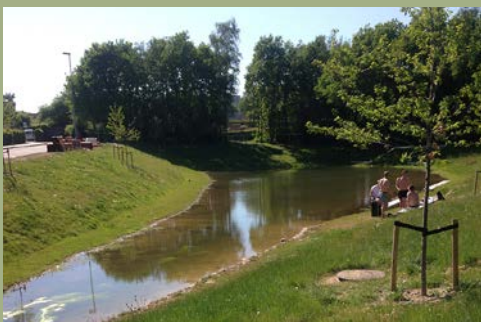
A rainwater reservoir in Risvangen with recreational possibilities. The water is retained when it rains heavily.
