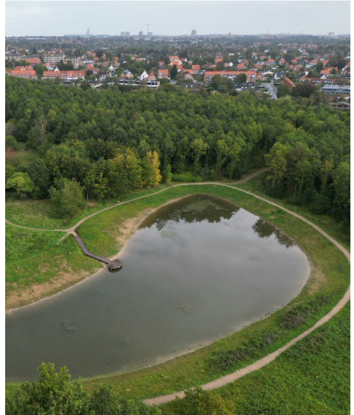
Photo: In Gellerup Forest, rainwater basins have been incorporated to create space for water.
