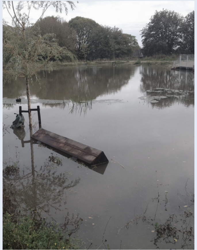
Photo: Stormwater pond at Klokkervej Åbyhøj, after October 3, 2023
