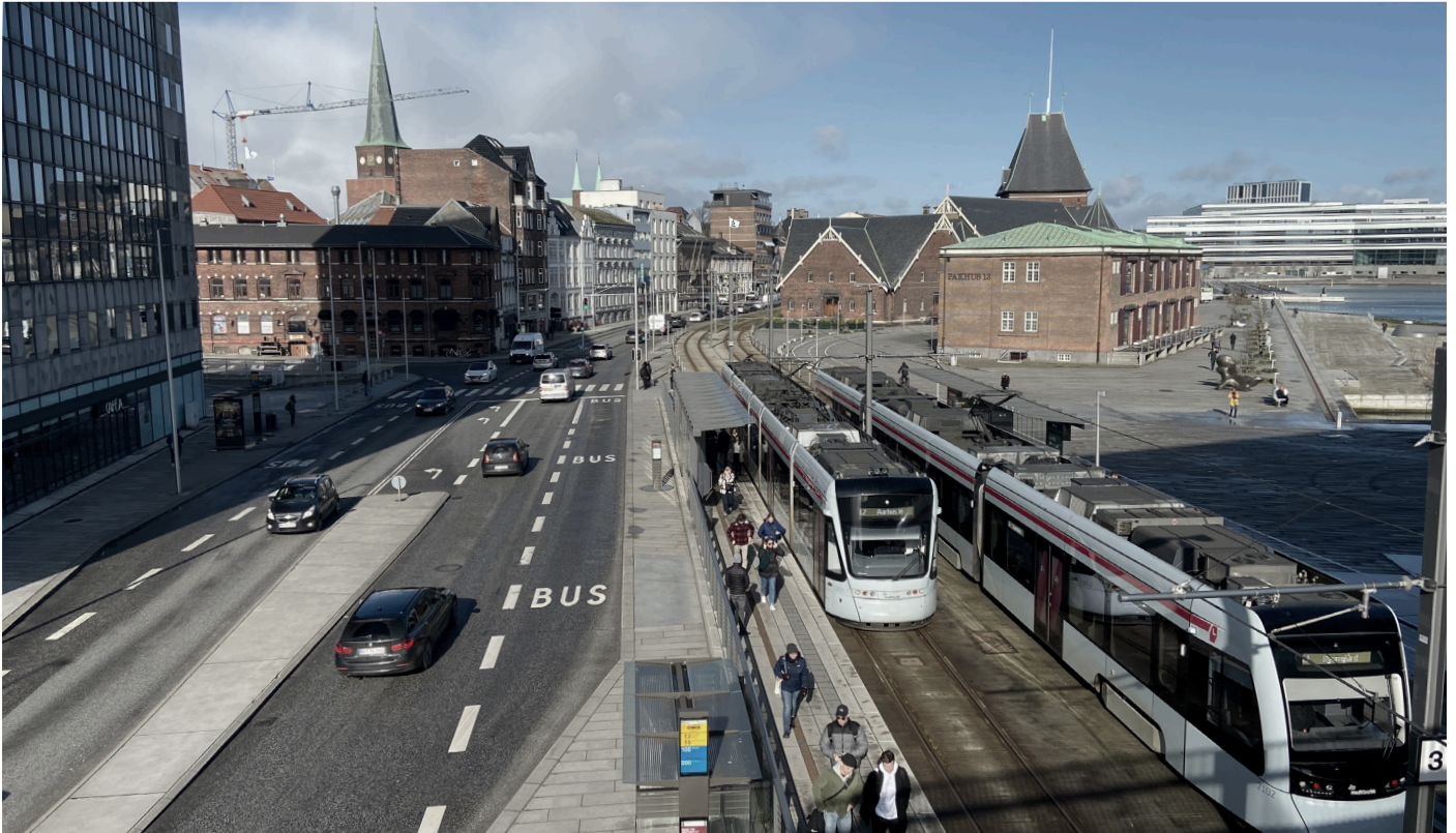
Photo: The light rail in Aarhus was established alongside the coastal road (Kystvejen) which functions as a high-water barrier from DOKK1 to Skolegyde, protecting the city center from rising sea levels.
