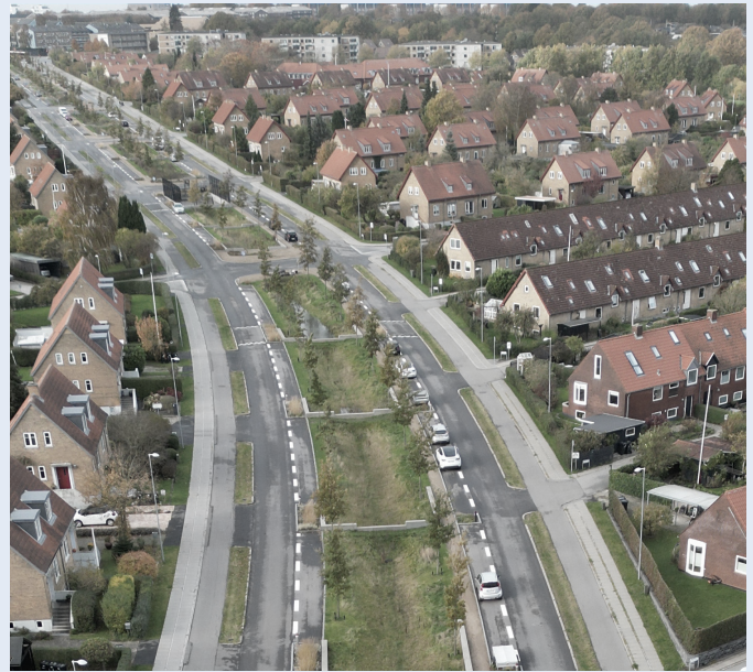
Photo: We are making good progress in adapting Aarhus to climate change and, in collaboration with Aarhus Vand (water utility), we have carried out several recreational adaptation projects. Here, Risvangen is shown, adapted to stormwater management in recreational areas.
