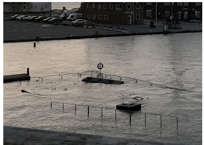
Photo: High water levels in Aarhus Bay in December 2023. Flooding of the lower plateaus around DOKK1 and water levels very close to the harbour pier's surface. The high-water lock was closed due to a high water level.
