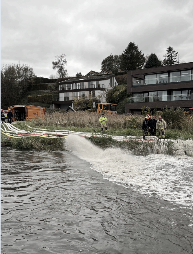
Photo: October 29. Aarhus Municipality and the emergency services were ready to pump water away from the river system in Egå with additional pumps at the high-water lock in Egå.
